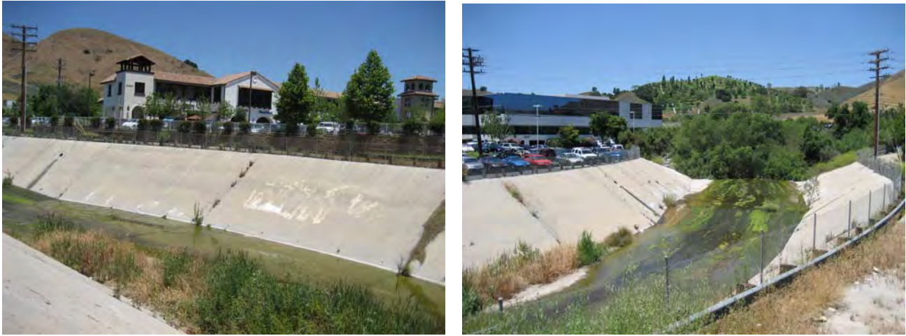
Concrete Channel built in 1977
