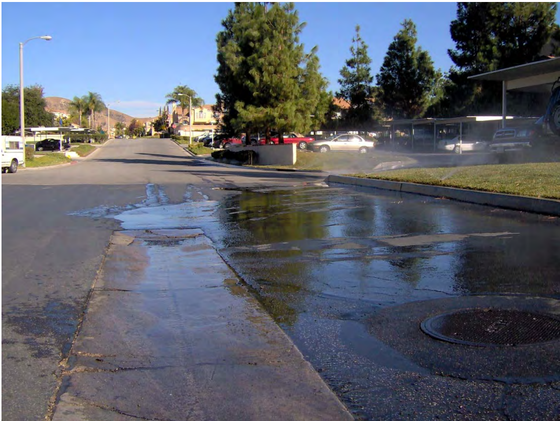
Image 3: Irrigation runoff at south end of Poppyseed lane entering a storm drain
